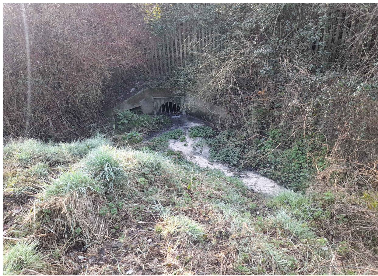
EXISTING STORM OUTLET
